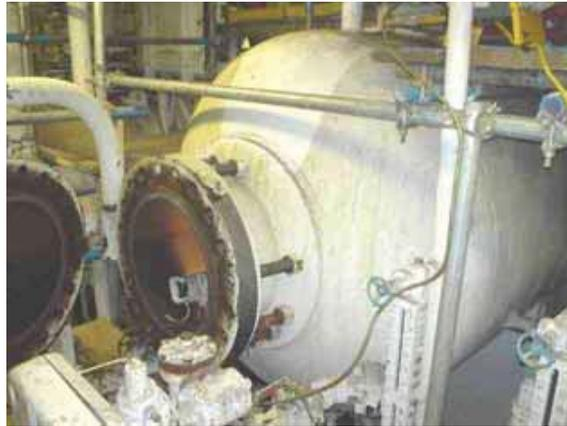
**Photo 6. One of the 2 separators where the sludge sample was collected**
