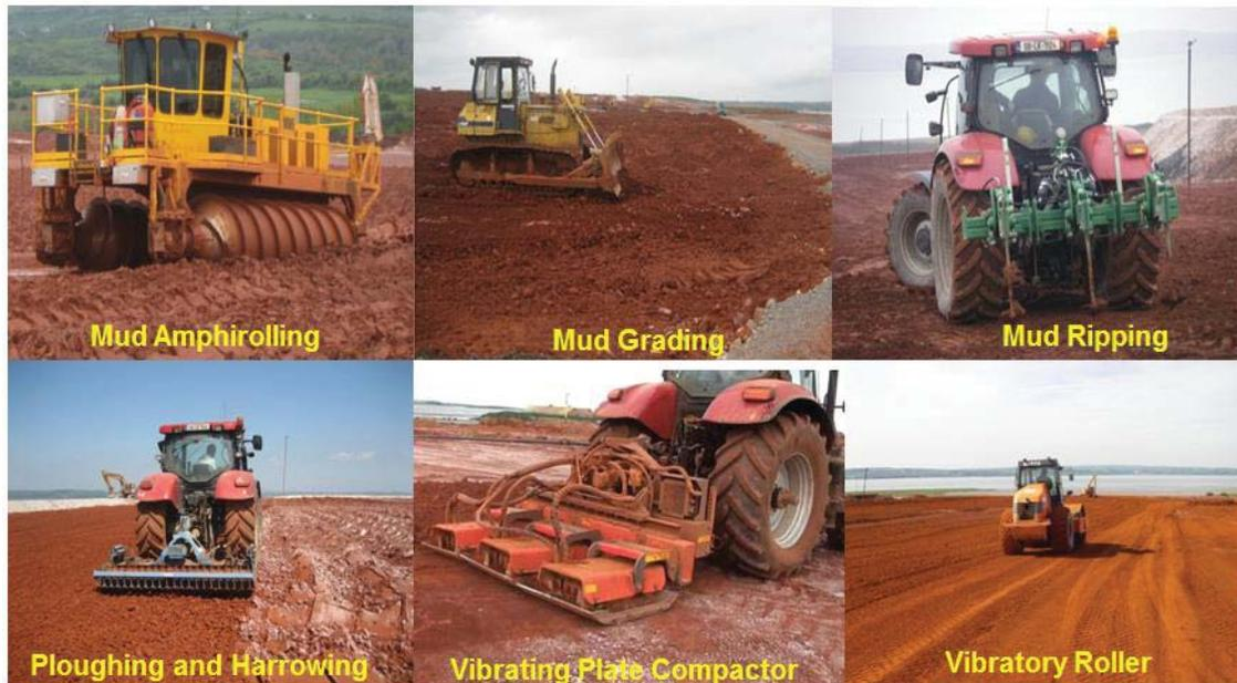
Figure 1: Bauxite residue farming and atmospheric carbonation process at RAAL
